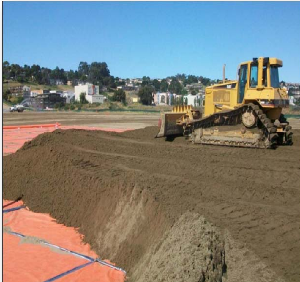
Installation of protective liner with soil cover
